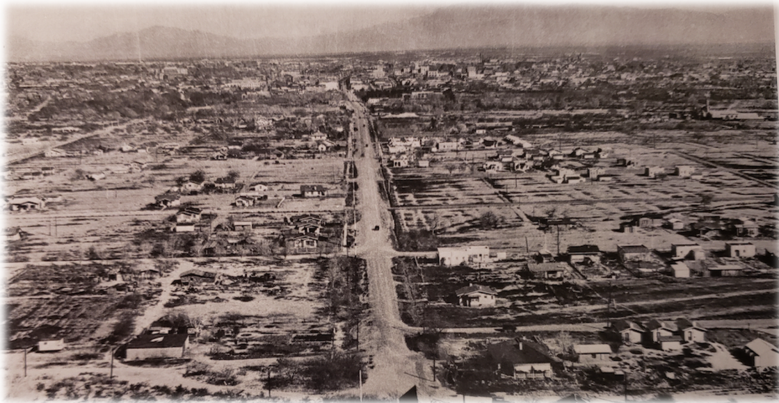
Fig 20 and 21. West Congress Street, looking east, as seen from the northern end of the Powderhouse Hill ridge located between Sentinel Peak and Tumamoc Hill. George Roskrige took the upper photo around 1890. A row of cottonwoods runs along the West Branch of the Santa Cruz which indicates this tributary of the Santa Cruz and therefore the Santa Cruz River must have been farther east than it is today. Today the West Branch is channeled to the main river channel south of Sentinel Peak. Currently, there would be no opportunity for the West Branch to pass between Sentinel Peak and the Santa Cruz River. The lower photo from the same perspective was taken in the 1930s by E. Ronstadt. Agriculture appears to have been replaced by low-density home sites. The Santa Cruz is still barely visible in the distance. The ancient flood plain had now evolved into an arid, sparse terrace above the river, ready for urbanization. 26
