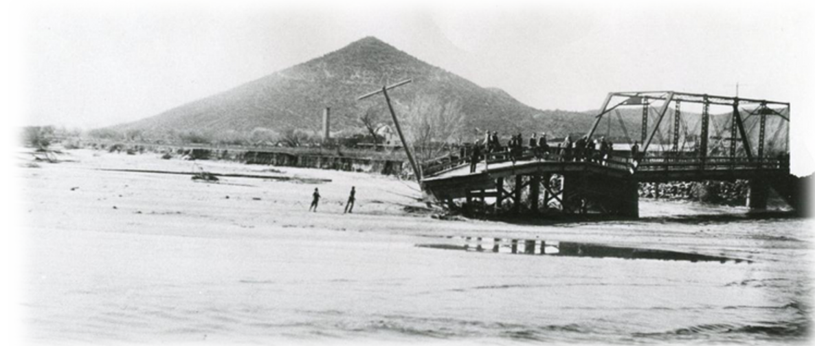
Fig 29. A bridge within sight of Sentinel Peak, likely on Saint Mary's Road, washed out in a 1915 flood adding to the west side's sense of disconnection. Is the smokestack on the shore part of the Tucson Pressed Brick Company? 48 (Photo from Arizona Daily Star)
