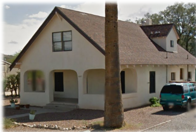
Fig 54. The exceptionally well-preserved two-story adobe house that Henry Schwalen purchased sometime after his 1905 arrival in Menlo Park. Like many of the homes of this period, it occupied a 20-acre or more parcel of land. The interior of this home contains a ‘truth window’, an opening that reveals an earlier adobe wall, from the core 1797 farmhouse. It is possible that this older dwelling is one of the only farmhouses in Carlton Watkins’s photograph of the Menlo Park flood plain taken from Sentinel Peak in the 1880s, page 31.
