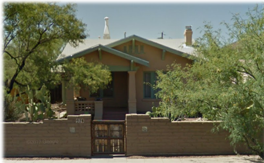
Fig 49. Bungalow with typical front gable, offset triangular porch and roof knee braces.
