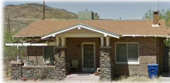
Fig 48. Example of a simple Bungalow with local Sentinel Peak basalt columns. There are several variations on this style. This design has a cross gable.
