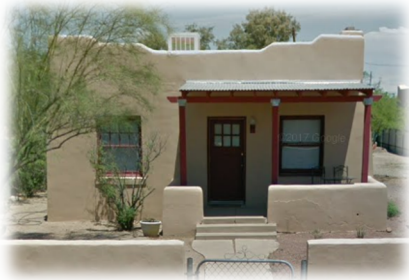
Fig 47. Example of simple Spanish Colonial Revival style home. Variations exist commonly with shallow pitched 'shed' roofs.
